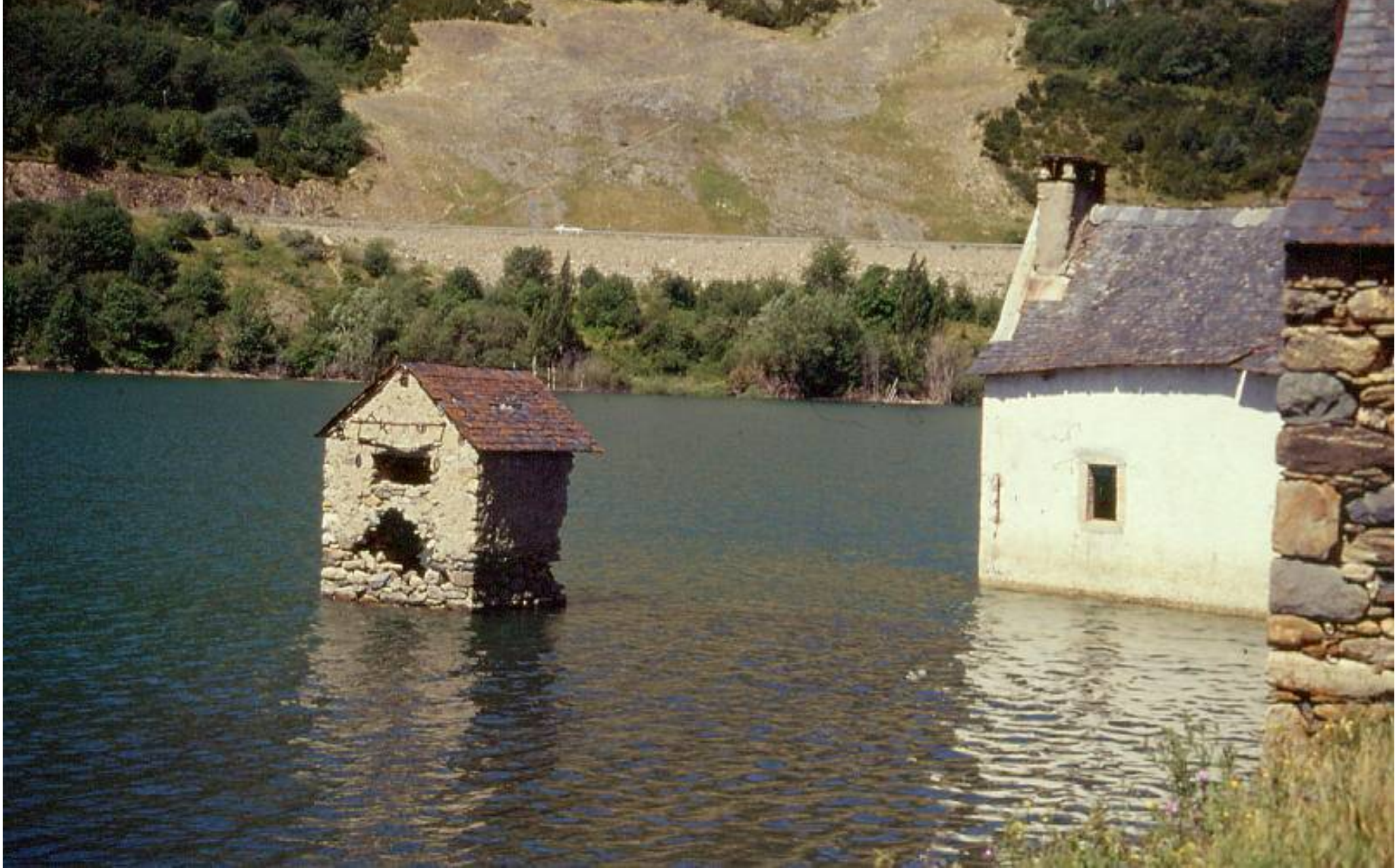
Flooded Village, Yeza Reservoir in Spain (1998). Now it is planned to heighten the dam
